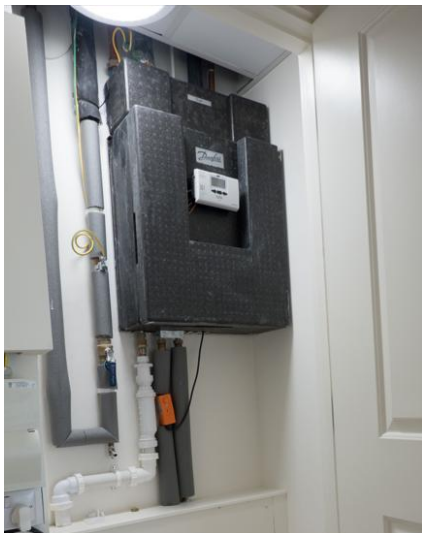
Fig 26 HIU with and without cover.
