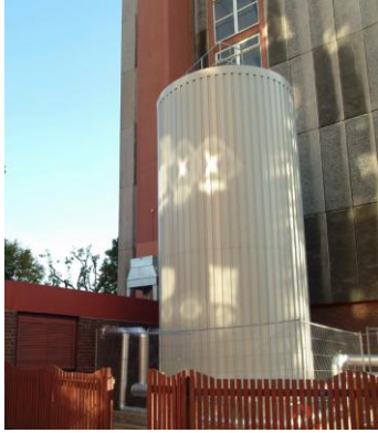
Figure 27 Example of thermal store of a size similar to that proposed – but the recommendation is for the store to be within the energy centre
